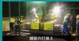
舗装の打換え
