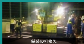
舗装の打換え
