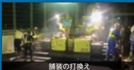
舗装の打換え
