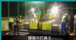
舗装の打換え
