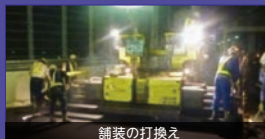
舗装の打換え
