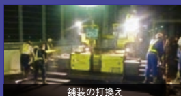
舗装の打換え
