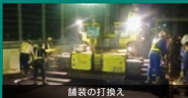
舗装の打換え
