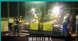
舗装の打換え
