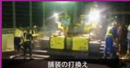
舗装の打換え
