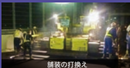
舗装の打換え
