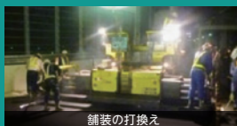
舗装の打換え
