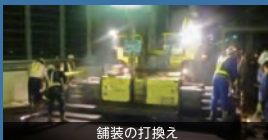
舗装の打換え
