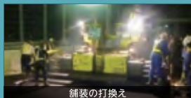
舗装の打換え
