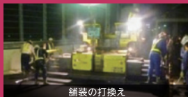
舗装の打換え
