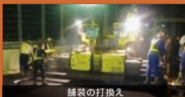
舗装の打換え
