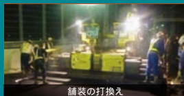
舗装の打換え
