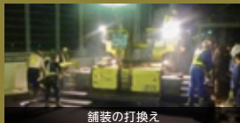
舗装の打換え
