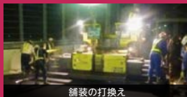
舗装の打換え
