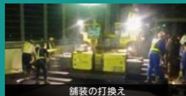
舗装の打換え
