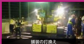
舗装の打換え
