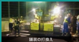
舗装の打換え
