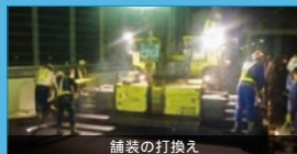
舗装の打換え
