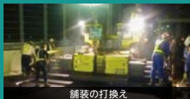
舗装の打換え
