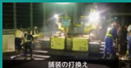
舗装の打換え
