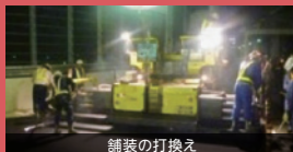
舗装の打換え
