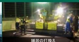
舗装の打換え
