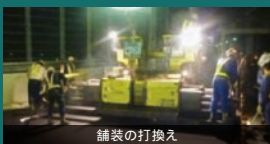
舗装の打換え
