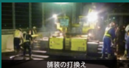
舗装の打換え
