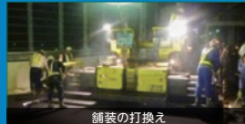
舗装の打換え
