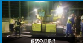
舗装の打換え
