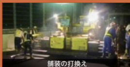
舗装の打換え
