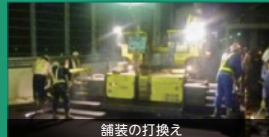
舗装の打換え
