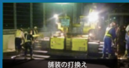
舗装の打換え
