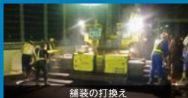
舗装の打換え
