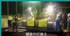
舗装の打換え
