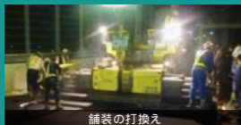
舗装の打換え
