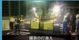
舗装の打換え
