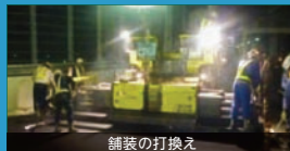
舗装の打換え
