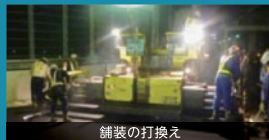
舗装の打換え
