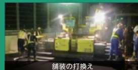
舗装の打換え
