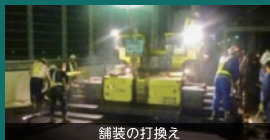
舗装の打換え
