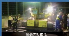
舗装の打換え
