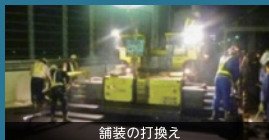
舗装の打換え
