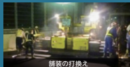
舗装の打換え
