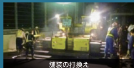
舗装の打換え
