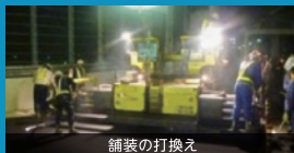
舗装の打換え
