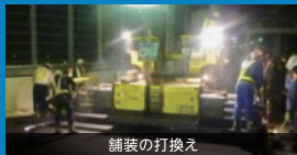
舗装の打換え
