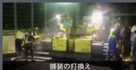
舗装の打換え
