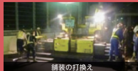
舗装の打換え
