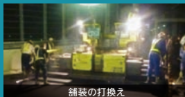
舗装の打換え
