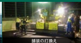
舗装の打換え
