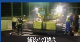
舗装の打換え
