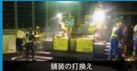
舗装の打換え
